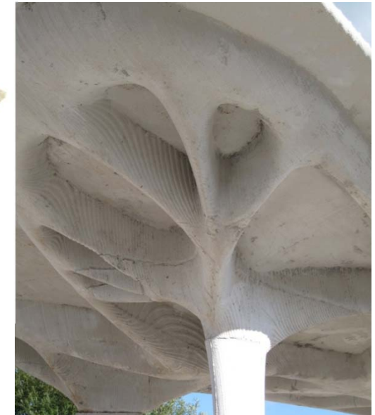
Concrete structure ( www.digitalcrafting.dk )
